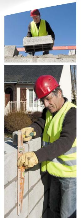
Stabilized Morbricks is a series of different grades of high quality premixed mortar batched in Lafarge's concrete plant, delivered to site ready to use. No addition of water or other raw materials is required on site.
