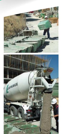
Stabilized MorPlast is a high quality plaster batched in Lafarge's concrete plant, delivered to site ready to use. No addition of water or other raw materials is required on site.
