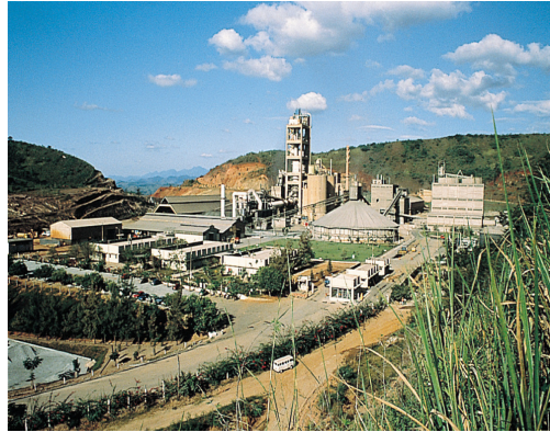
Matozinhos cement plant, Brazil
