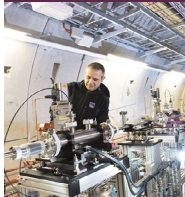
High-performance concrete by LafargeHolcim for the tunnels of the European XFEL - (Photo: European XFEL)
